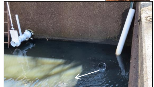
A submersible pump on a timer was used to refill the basins from the catch basin after zooplankton release.
