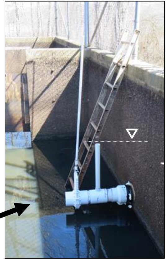
An airlift pump chamber was installed to circulate water from Cell 4 to Cell 1.
