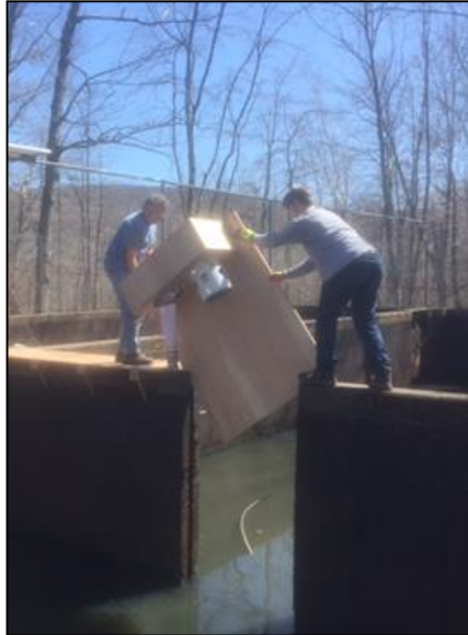
A walkway was installed to provide access to all four Cells.
